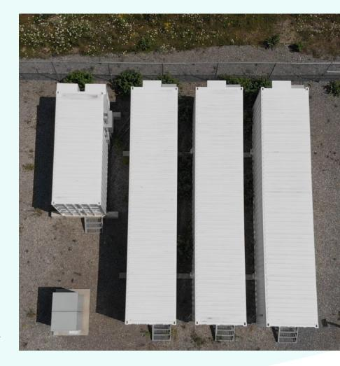
Convergent's 0.5 MW / 3 MWh system is comprised of three 40' Energy Storage Modules and one 20' Power Control module.
