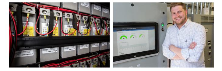
The system was integrated and warranted by Lockheed Martin, using over 1,800 VRLA batteries from C&D Technologies.
